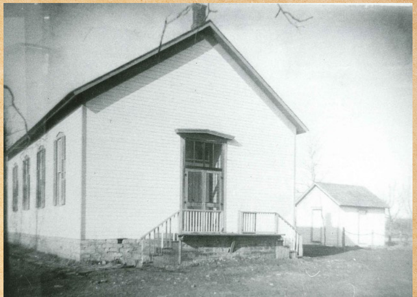
The First Emmaus Building
